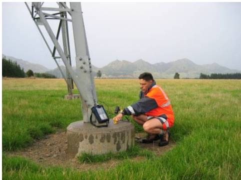
Checking tower leg foundations at remote stations in New Zealand using the TDR2
