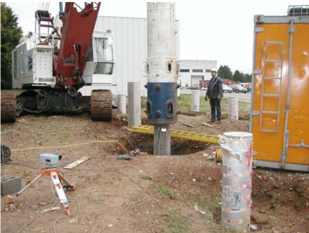
Fig 14. Guide tube for 4 tonne mass.
