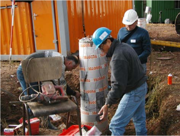
Fig 13. Three sets of instruments being attached to pile top
